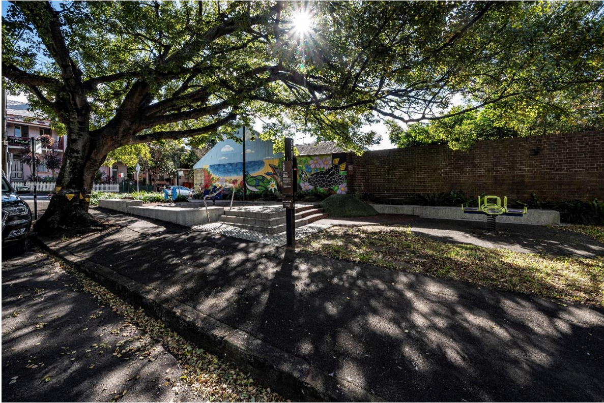
Existing playground in the park, looking north from Glebe Street. Play equipment is at the end of its useful life and soft fall is worn and separating at edges. Playground is well shaded from the existing tree. Small area of turf in poor condition.
